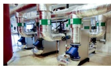
SWEP's ETS: 3x6MW units connected in parallel.
